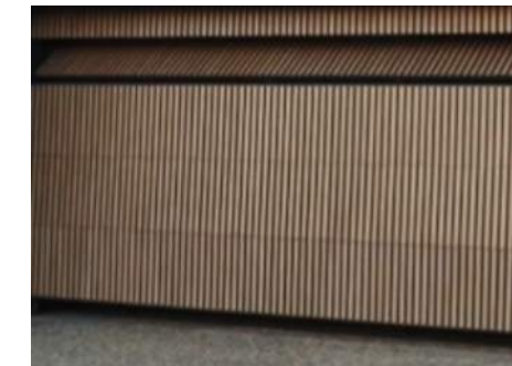
L - POWDERCOATED ALUMINIUM PANEL LIFT GARAGE DOOR
