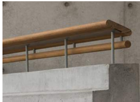
E - TIMBER HANDRAILS
