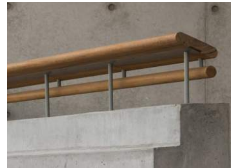
E - TIMBER HANDRAILS
